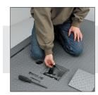
Maintenance inspection plate in the deck to allow for maintenance above the dock.
